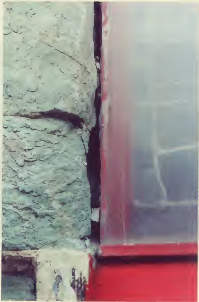
West Façade of Church Building (C) window detail
